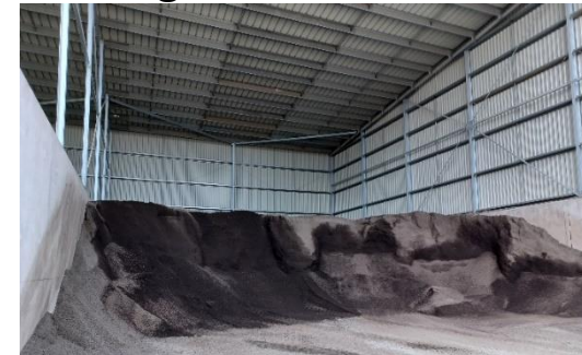
Storage of RAP
