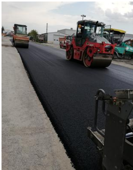
Fig.13. Built-in AC 16W
